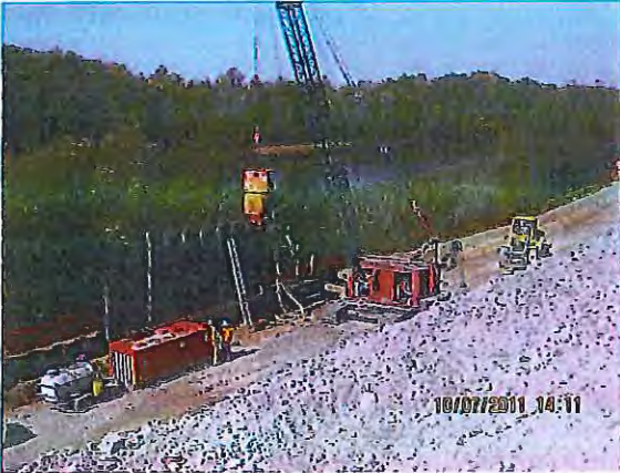
◀ Installation of the Waterloo Barrier Groundwater Barrier System
