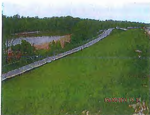
◀ Looking north along the west slope. Regraded and capped slope, Waterloo Barrier, newly installed groundwater monitoring wells, security fencing and surface water controls
