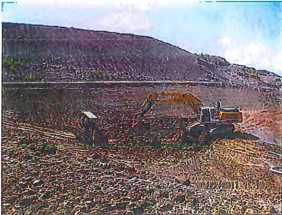
◀ Site remediation and preparation for engineered leachate collection pond
