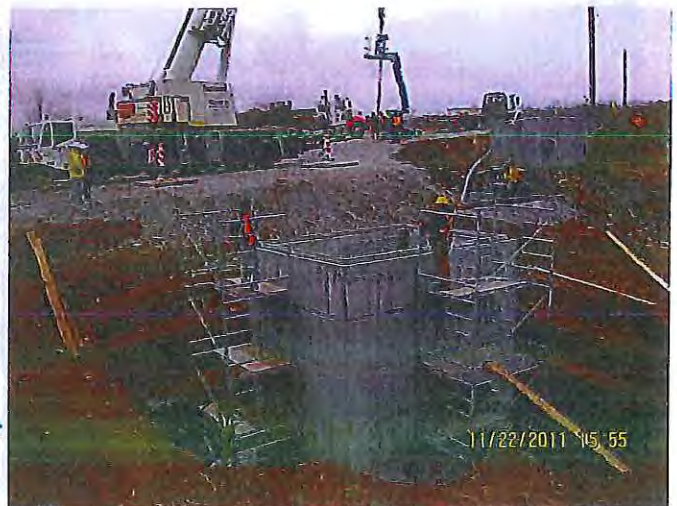
▶ Construction of the new leachate pump station (Pump Station PS1)
