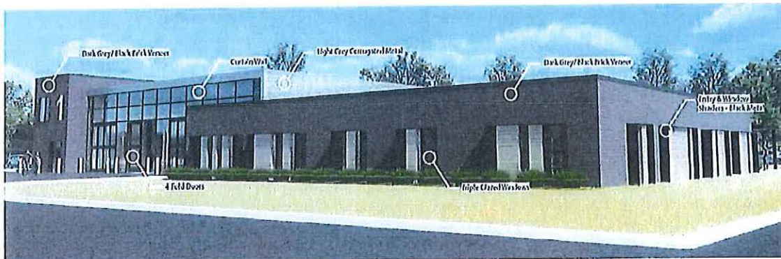
View of Station 1 – looking at front of building from East Main St. (South side of bldg.)
