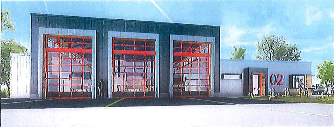
Station 2 – View from King St. (East side of bldg.)
