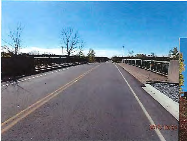
Nidel's Bridge – looking north
