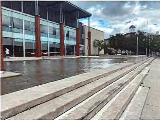
Accessibility - Reflecting Pool Creates a Barrier to Street and is a Maintenance Concern
