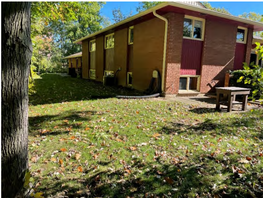
Figure 14. Roof top water is an extraneous addition of water into the seasonal pool area within the subject lands. Pipes were found as above (top) and from the back of the house (bottom) that discharge overland into the woodland's seasonal pool feature.
