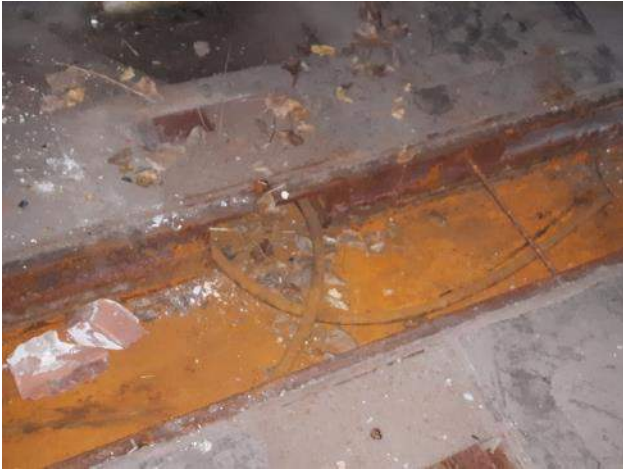
Photo 7: View of the trench drains in workshop area of Site Building-X.
