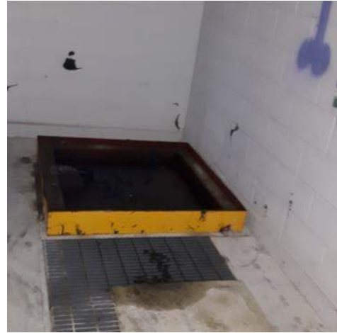
Photo 8: View of the oil pit in southeast portion of Site Building-X.
