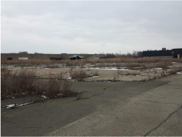
Photo 1: View of the Site buildings (facing northeast).
