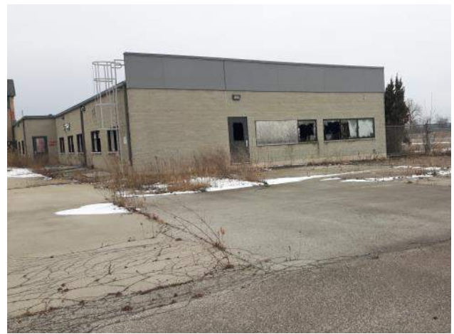
Photo 2: View of the northwest portion of Site Building -X (facing southwest).
