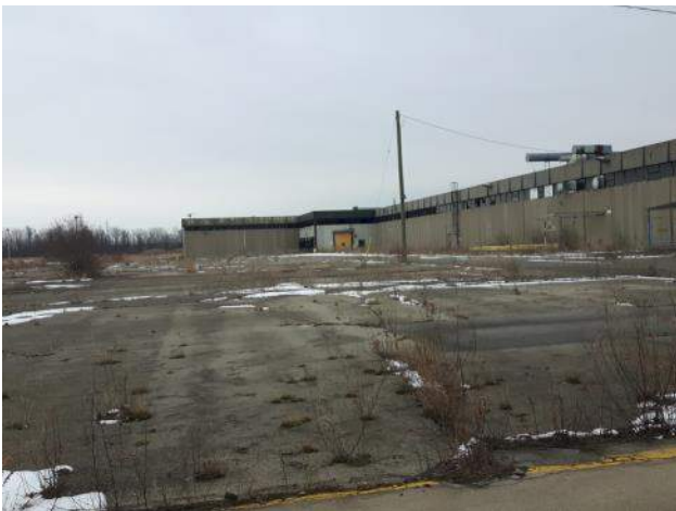
Photo 3: View of north portion of Site Building-Z (facing east).
