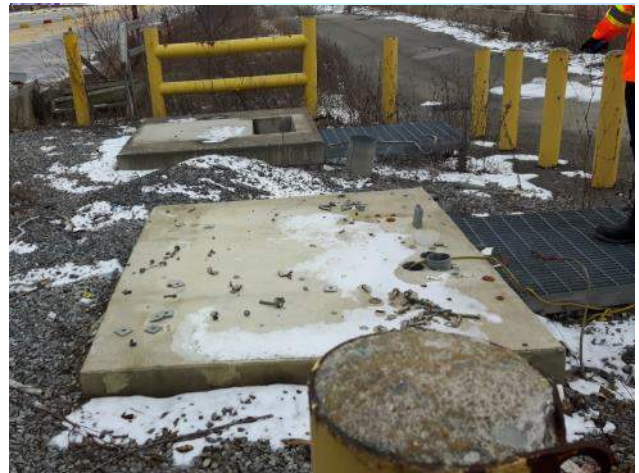
Photo 10: Two USTs southwest of Site Building-X (facing west).
